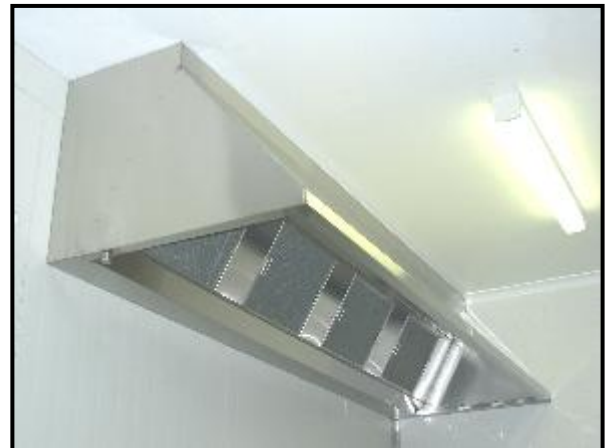
Mechanical exhaust canopy
