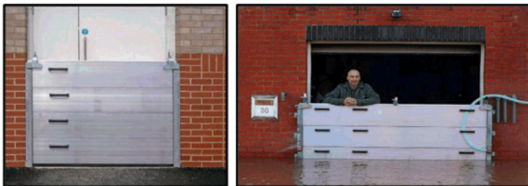
Figure 4-7 L-Series Modular Demountable Flood Barrier (Flood Control International, 2015)
