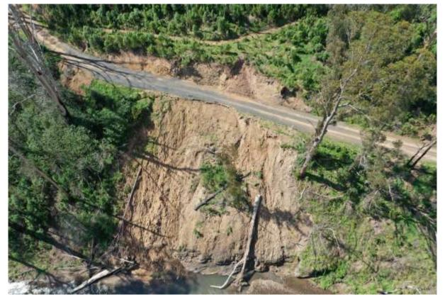
Figure 5 - Upper Middle Creek Road landslip October 2021 with temporary works completed
