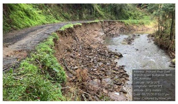
Figure 4 - Site 33, Morwell River East Branch Road, 23 June 2021 river erosion
