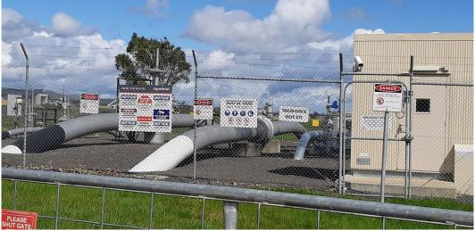
Plate 2: High pressure buried oil pipeline compound in southeastern corner of the site
