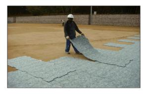
Photo 41: Prefabricated Shockpad being laid (Source: TEAM Sports)
