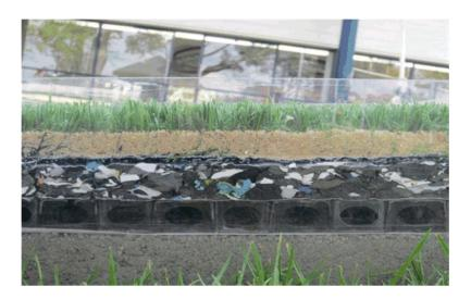
Photo 43: Example of horizontal drainage cell under shockpad (Source: Wayne Stuart - City of Swan, WA)
