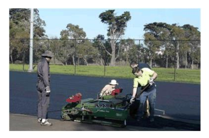
Photo 42: Insitu Shockpad being laid (Source: Polytan)
