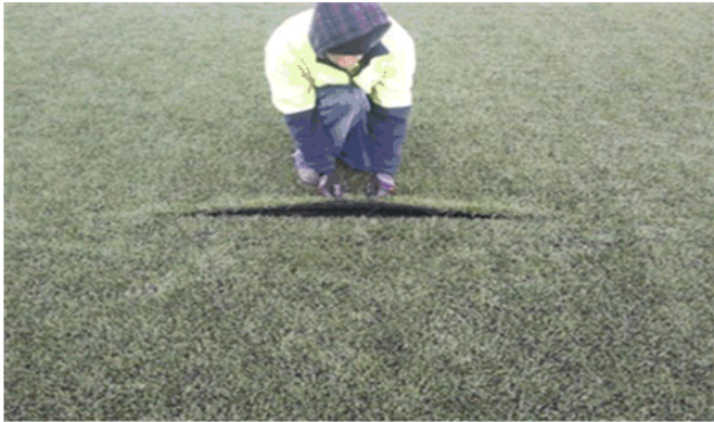
Photo 34: Example of seam failure
