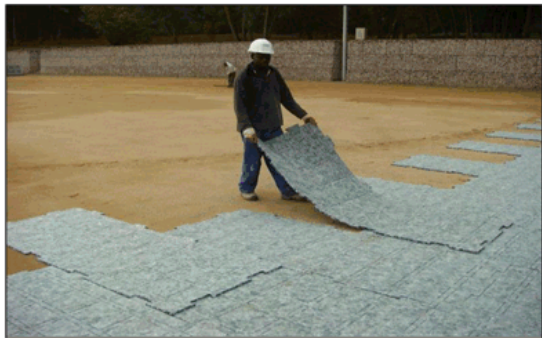
Photo 41: Prefabricated Shockpad being laid (Source: TEAM Sports)
