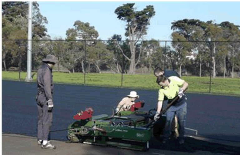
Photo 42: Insitu Shockpad being laid (Source: Polytan)
