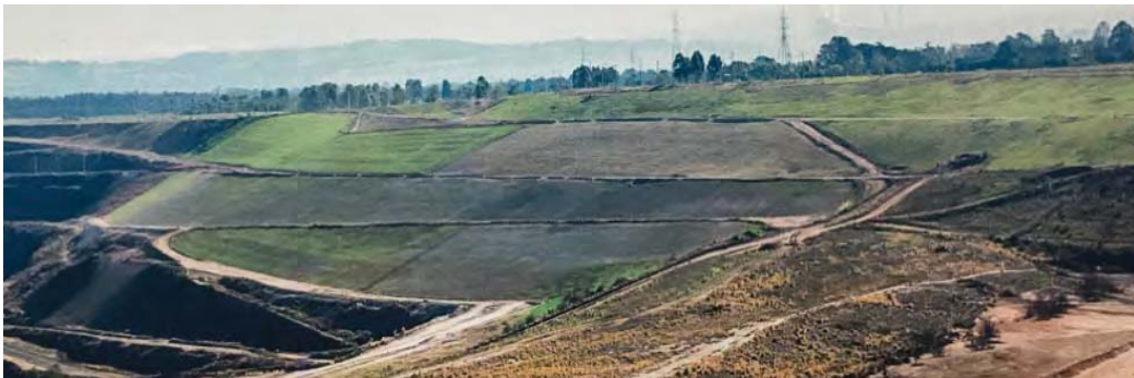
Image 8: Rehabilitation works undertaken to the Hazelwood mine (northern batter).
