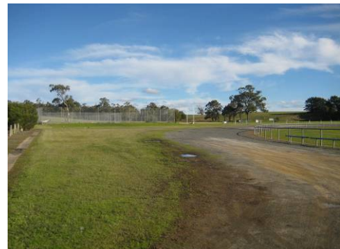
Figure 21: Unsealed surface around south oval
