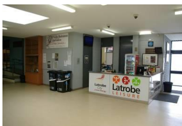
Main entry, control / reception counter. Counter not catering for wheel chair access by patron/ player.
