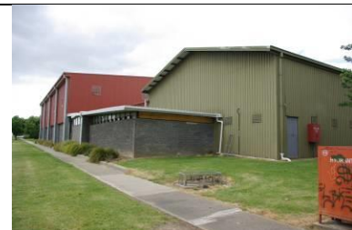
Existing multi-purpose hall with community meeting rooms – overall in fair condition.
