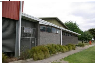
Junction of existing multi-purpose building with show court.
