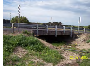
LTB035 Crinigan Road MORWELL
