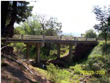
LTB085 Glengarry North Road GLENGARRY NORTH
