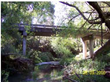
LTB200 Livingston Road BOOLARRA SOUTH
