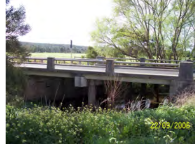
LTB040 Crinigan Road MORWELL
