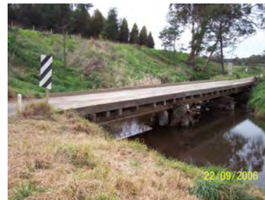
LTB050 Downies Lane TRARALGON SOUTH
