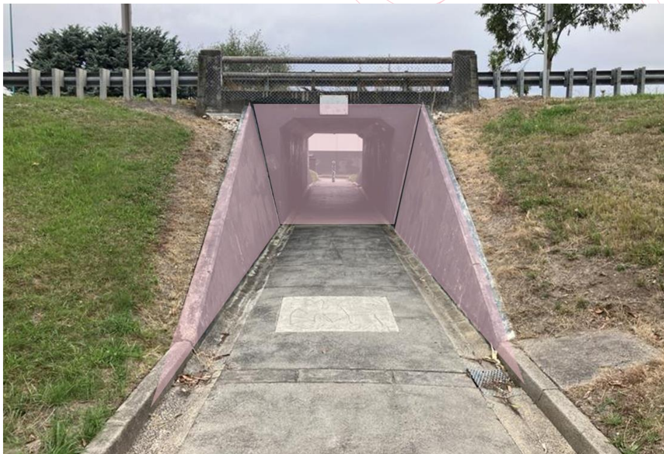
Above: photo of the underpass, west end, tunnel and side abutment walls highlighted in pink
