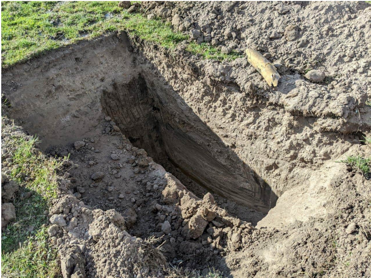
Photograph 23: View of TP08. Trace fill inclusions were observed within test pits within the filled area.
