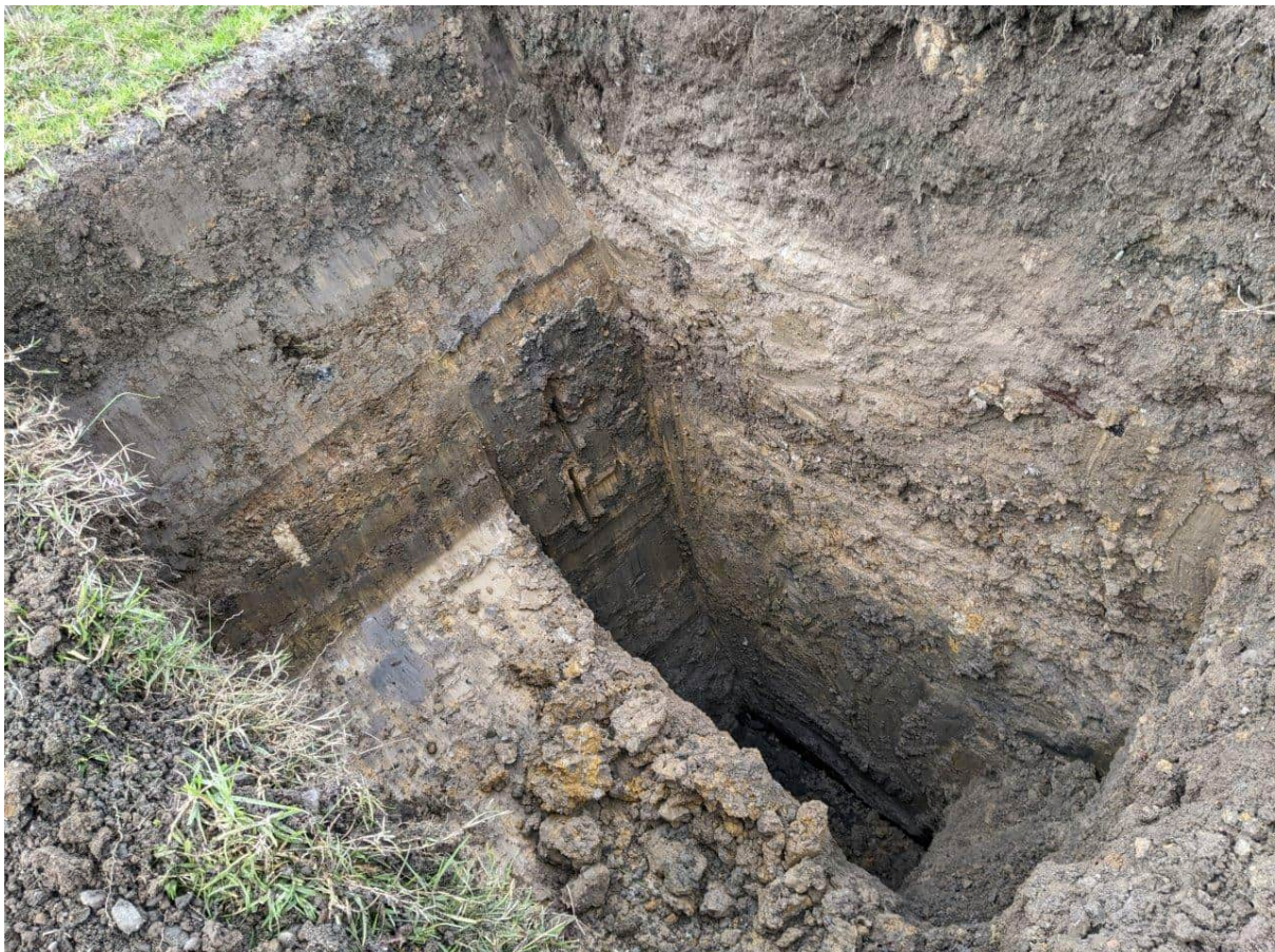
Photograph 18: View of TP03. Trace fill inclusions were observed within test pits within the filled area.
