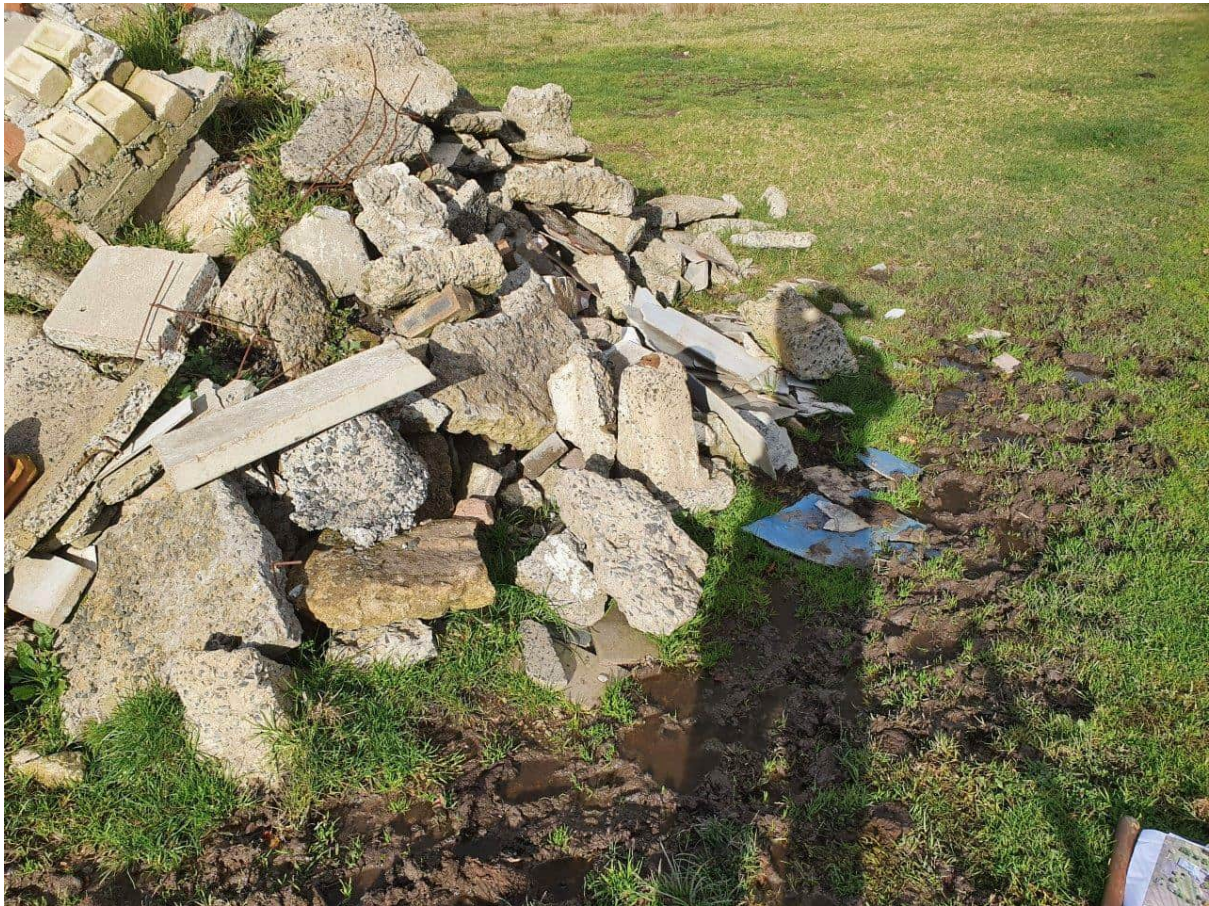
Photograph 15: View of a stockpile of rubble (concrete, bricks, cement sheet (non-ACM?)) in the homestead area of site.
