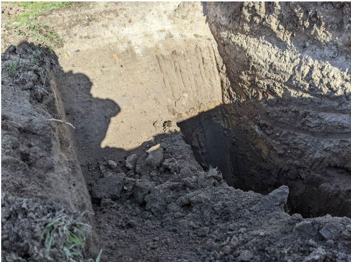
Photograph 22: View of TP07. Trace fill inclusions were observed within test pits within the filled area.
