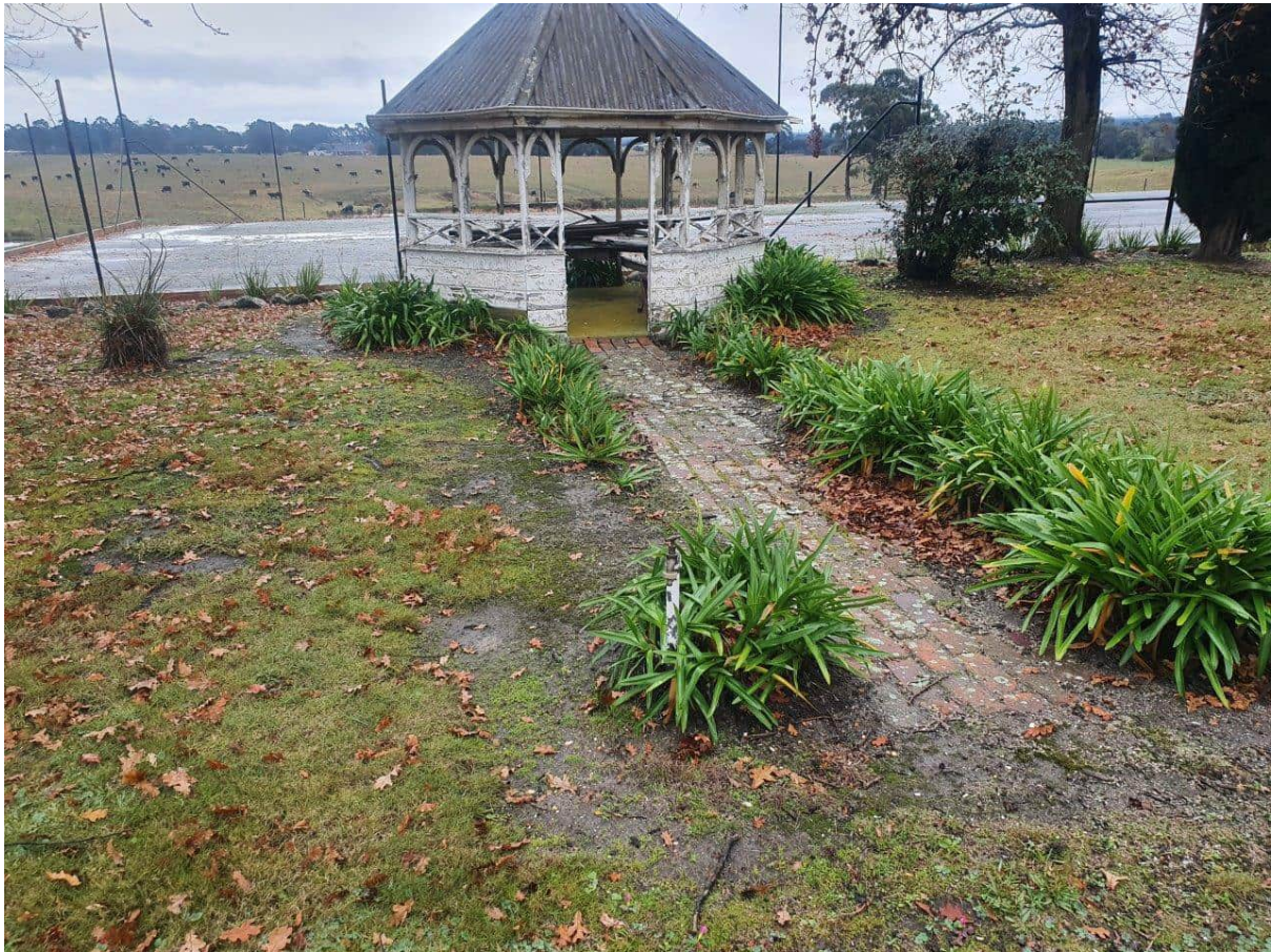
Photograph 5: View of a gazebo and tennis court in the homestead area of the site. Potential lead paint was observed on the gazebo exterior.
