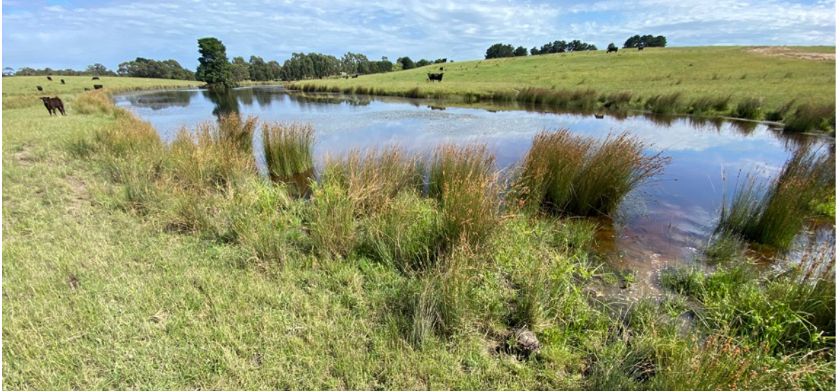
Photo 6 Dam 1 looking downstream northwest
