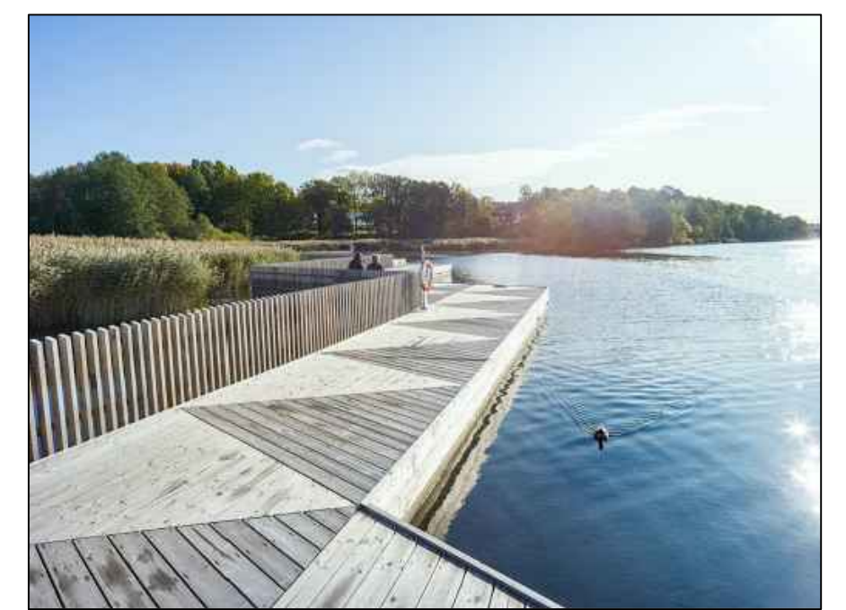
6 Boardwalk through new wetland area
