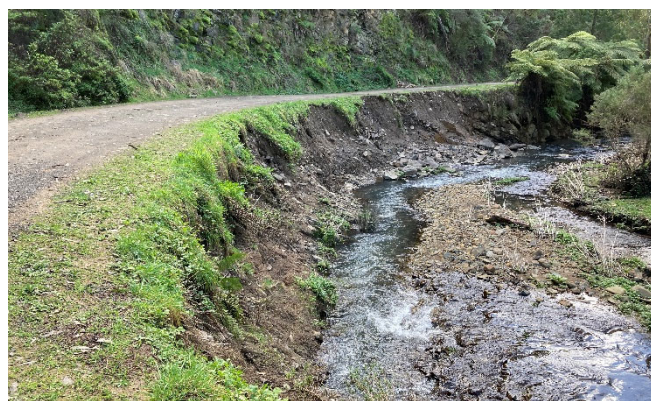
Figure 3 - Flood damage on Traralgon Creek Road during 2021
