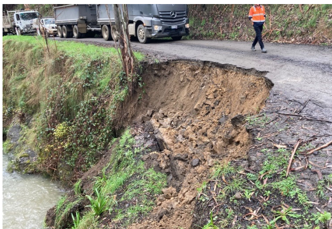
Figure 1 - Landslip damage holding up traffic on Traralgon Creek Road soon after the August 2022 storm
