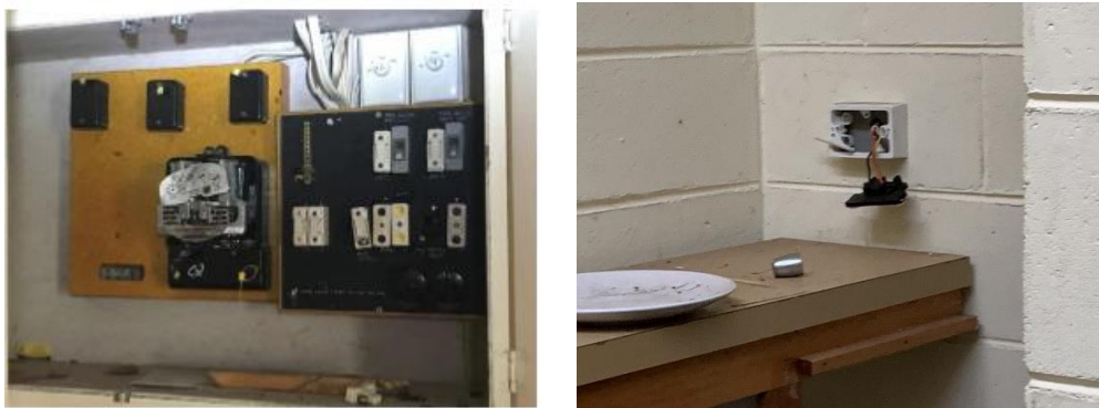
Figure 5 Pavilion Meter Box and Damaged Power Point
