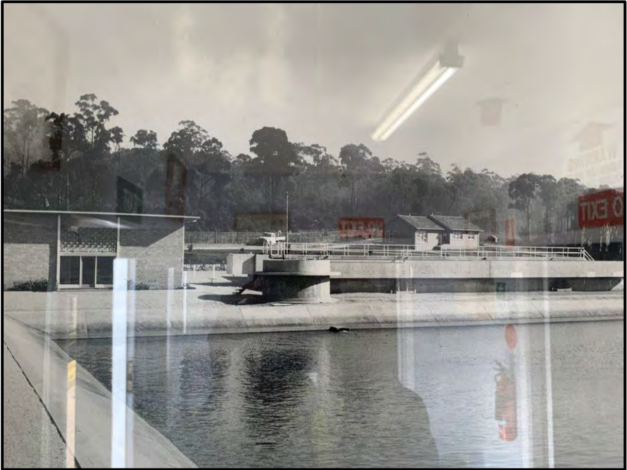
Figure 3: 1961 Photograph showing the Newly Constructed Treatment Plant with the Operators House at the Rear
