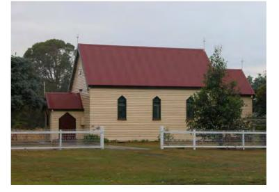
**DESCRIPTION** St Columbkille's is a simple Carpenter Gothic Church with typical detailing including lancet windows with diamond pattern leadlight glass in the side elevations. It has a small projecting gabled porch with a lancet door and a gabled vestry at the rear. There is a small circular vent in the front elevation and there a small crucifix is placed at the apex of each gable.
