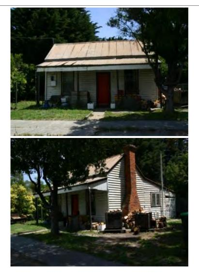
**DESCRIPTION** 11-13 Janette Street is a late nineteenth century weatherboard cottage, with a gabled roof, rear skillion and a single external brick chimney. The front door is unusually placed slightly off centre and is flanked by double hung timber windows with 6-paned sashes. The verandah is a skillion in form, with shaped posts. The timber floor has been replaced with concrete. The verandah is a skillion in form, with shaped posts. The timber floor has been replaced with concrete.
