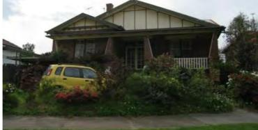
**DESCRIPTION** The house at 96 Princes Street, Traralgon is a brick California Bungalow set high above the street. It has an unusual roof form with wide gables on at least four sides. It incorporates tapered piers on a small gabled bay with extensive render as a detail and paired windows with four-paned upper sashes. The house is well detailed, reflecting the skills of the builder. It appears substantially intact externally.
