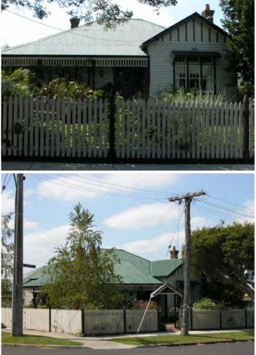
**DESCRIPTION** 70 Moore Street is a good example of an asymmetrical Edwardian villa, with the roof extended to form a wide return verandah ('homestead' roof form). Notable features include half timbering to the gable end, six-pane sash windows, pressed metal hood over a triple light window, entry door with side and highlights, timber 'ladder' fretwork and curved brackets on the verandah, and two brick chimneys, one with a terracotta pot. (quite similar in form to that found on 6 Moore Street).
