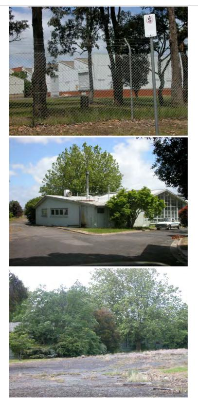
**DESCRIPTION** The former La Mode factory is a post-war industrial complex. The factory comprises a saw-tooth factory building with smaller gabled buildings adjoining, which is attached to an office and administration wing. The factory building is clad in corrugated iron with brick to the lower walls. The office is 'T' shaped in plan and has a gabled roof with prominent eaves and extensive glazing in the walls, which are otherwise constructed of brick. There is a small gatehouse with skillion
