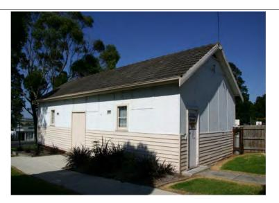
**DESCRIPTION** The former H.J. Saunders Sawmill Social Hall is a small weatherboard and fibro-clad utilitarian building located in front of the Tyers Community Hall (Refer to separate citation in this Study). It has a gabled roof, reclad with cement tiles. The fibro walls are strapped. The front door is timber and windows are simple double-hung sashes.
