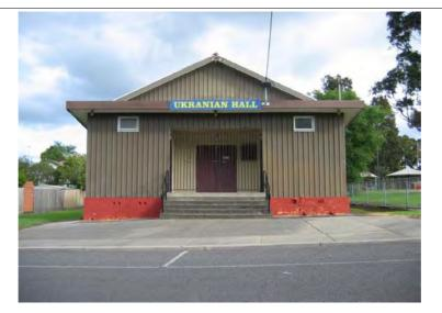
**DESCRIPTION** The Ukrainian Hall is a small utilitarian rectangular hall clad in steel decking. It has a gabled corrugated iron roof, with a reverse skillion roof to the projecting entrance. The building is a painted brick plinth. The large square six-paned windows in the side elevation are covered with wire mesh. Steps lead up to the recessed front entrance, which is flanked by two small square high set windows. The hall is setback from the street behind a concrete paved area.
