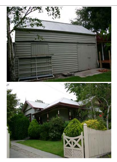
**DESCRIPTION** 'Danora' is an Edwardian villa with some Queen Anne details. While some alterations have been made many of original details remain. The form consists of two gable roofed sections projecting at right angles to each other with an equal-sided corner verandah between these bays. The three main windows are original, including the triple box window to the east with coloured highlights.
