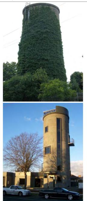
DESCRIPTION The Traralgon Service Reservoir or water tower is constructed of reinforced concrete. It is round in plan and approximately twenty metres high.
