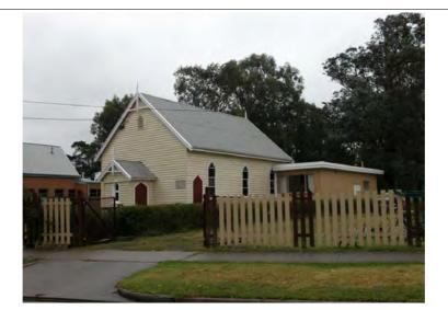
**DESCRIPTION** The Glengarry Uniting Church is a simple Victorian Carpenter Gothic church with typical detailing including lancet windows in the side elevations and a small projecting gabled porch with a pointed arch door and a small lancet window.
