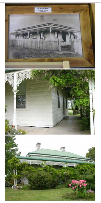
**DESCRIPTION** The homestead at 'Burn Brae' is a simple late Victorian Italianate villa, with verandahs on two sides, and a hipped roof, now clad in colourbond. Of typical design, form and layout, the building is notable for its internal and external cladding material: Both the exterior and interior walls are covered with pressed metal sheeting in a variety of ornate patterns. The external cladding simulates rusticated stonework and is believed to be a product produced by Wunderlich, which
