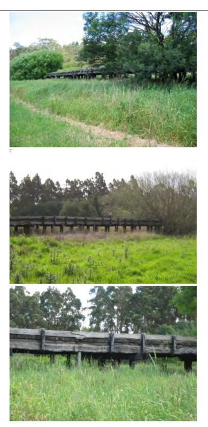
**DESCRIPTION** The Tyers Road (Bluff) Causeway Bridge is a low-level all-timber bridge of twenty-five spans, with a total length of 166 metres. According to the National Trust of Australia (Victoria):
