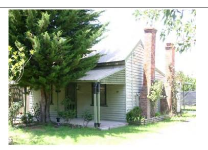
**DESCRIPTION** 10 Janette Street is a timber cottage, with a gabled roof, rear skillion and pair of external chimneys. The windows are double hung sash The verandah retains a scalloped valence on the east side. The building is, externally, relatively intact. The verandah floor has been replaced in concrete.
