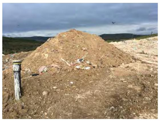
Photograph 9: Above cell 5 tipping face with stripped back cover and LFG well (looking south-west)
