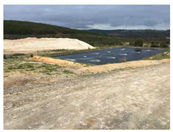
Photograph 13: Leachate Pond 2 with 9 of 10 aerators working (looking SW)
