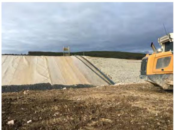
Photograph 7: Cell 5 South-west corner with gravel on side liner, leachate level monitoring point and leachate inspection line – adjacent Cell 4 (looking south)
