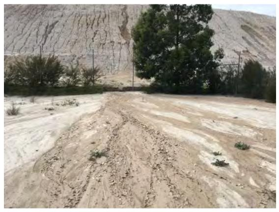
Photograph 23: Sediment from clay stockpile entering Stormwater Pond 2 (looking east)
