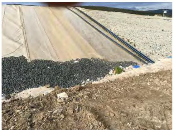
Photograph 8: Cell 5 South-west corner with gravel on side liner, leachate level monitoring point and leachate inspection line – adjacent Cell 4 (looking south)
