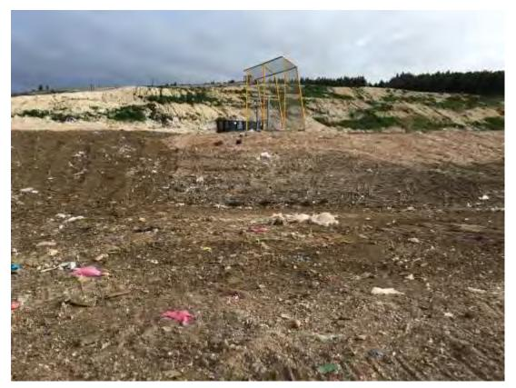
Photograph 2: Cell 5 north-north-west of tippling face with litter net and Cell 4 intermediate cover on batter (looking WNW)
