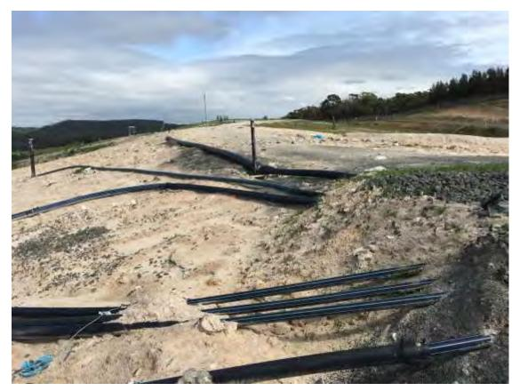
Photograph 28: LFG Inlets to Cell 4 manifold – Line 2 is temporary horizontal system in Cell 5
