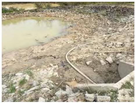
Photograph 20: Stormwater Pond 1 being cleaned – RO discharge temporarily diverted to Stormwater Pond 2 (looking south-west)
