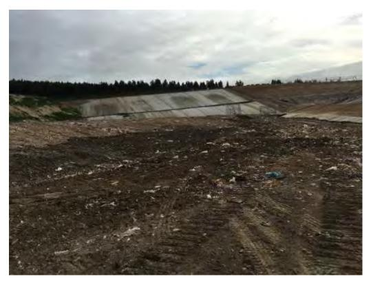
Photograph 4: Cell 5 with litter nets within cell and in north-west corner and waste through cap and staining on geotextile (looking NNE)
