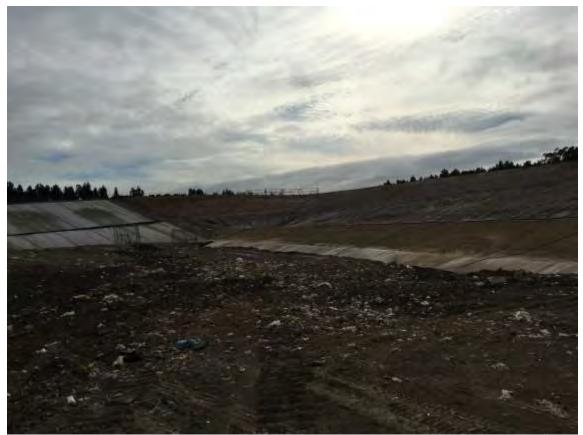
Photograph 3: Cell 5 north with daily cover, litter nets within Cell and in north-west corner and waste through cap (looking north-east)
