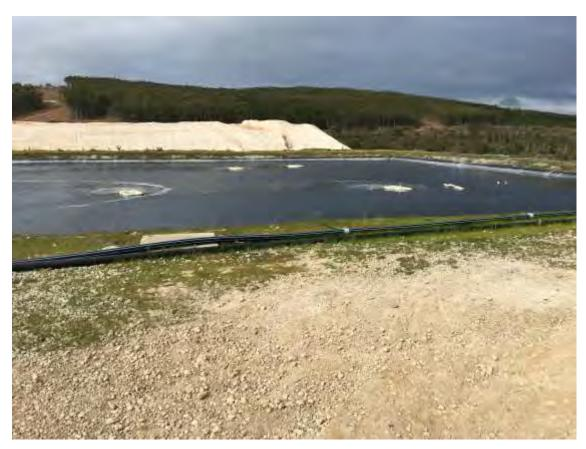
Photograph 15: Leachate Pond 2 near freeboard with fire-fighting pipeline C (looking south)
