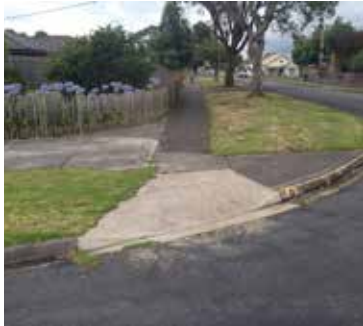
SINGLE RAMP- RECONSTRUCTED
